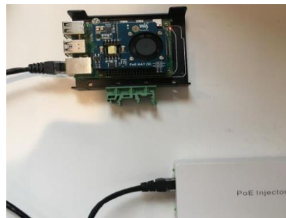
Fig. 11: Completed data & power configuration for single-cable operation of the microcomputer
