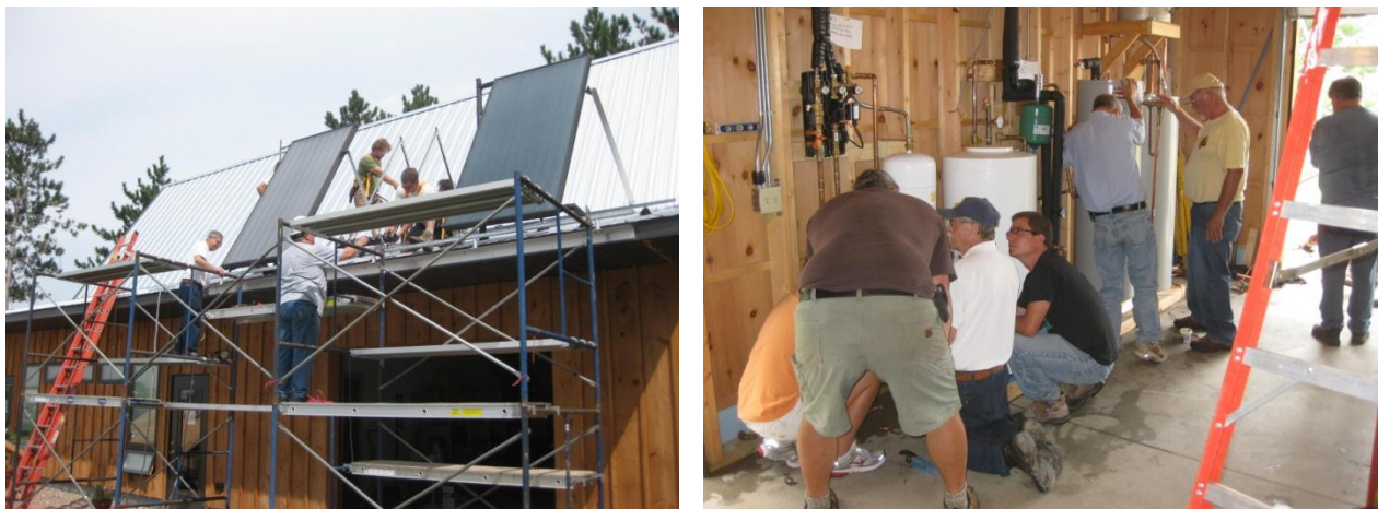
Figure 3. Instructor training includes hands-on installations of solar thermal systems.
