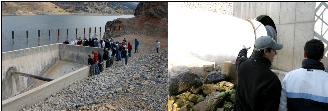
Figure 3. Dam field trip (A: service spillway intake and B: discharging fixed-cone valve).
