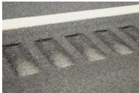
Figure 3. Rumble Strip on a Roadway [Safe Roads 2003]
