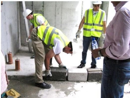
Picture 4: Under the supervision of Mr. Yabroudi, internship participants are learning how to build a masonry blockwall.
