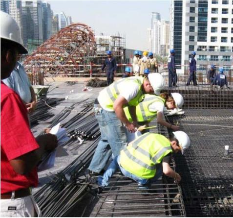
student interns are tying rebar at a construction site.
