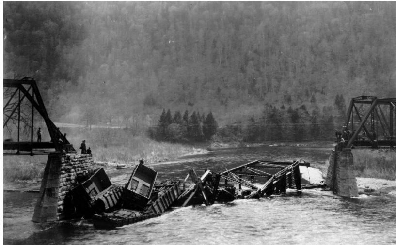
Fig. 1. Middle span collapse of the Fish’s Eddy Bridge in 1897. (DeForest Douglas Diver Railroad Photographs #1948. Division of Rare and Manuscript Collections, Cornell University Library.).
