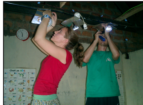
Figure 2: Students installing solar-powered lighting system.
