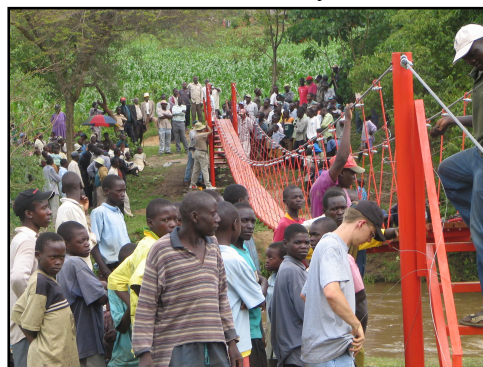
Figure 3: Construction of pedestrian bridge.
