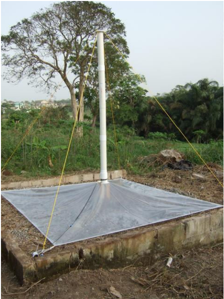
Figure 7: Small scale solar chimney in Ghana.
