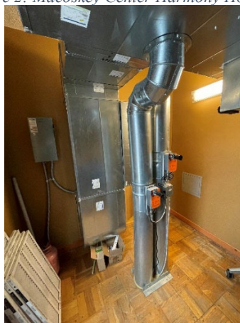
Figure 3: Harmony House geothermal ventilation ducts (left) and circulation pump (right)
