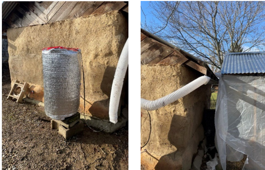
Figure 5: Chicken waterer (left) and gutter connection (right)
