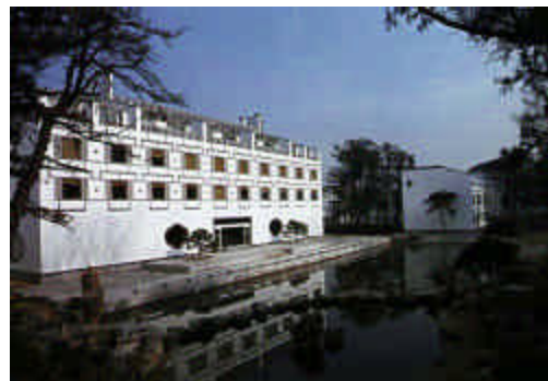
Figure 14: White Stucco on Exterior wall ( www.images.google.com )
