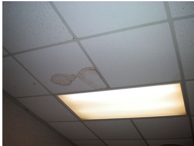
Picture 1: Acoustic tiles on the first floor
