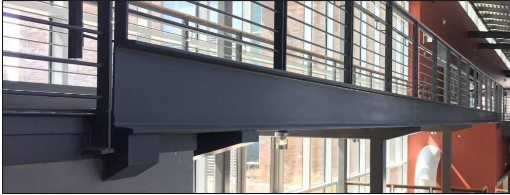
Figure 11. Pedestrian bridge with MC12x30 beams, looking west.
