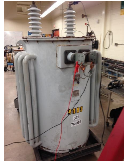
c. Low-voltage winding to high-voltage winding and to ground
