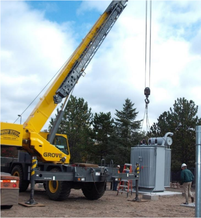
Figure 1. Placing the 2500kVA Transformer
