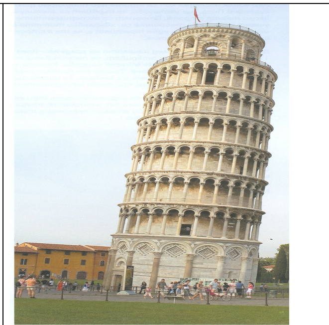
Fig. 2: The Leaning Tower of Pisa
