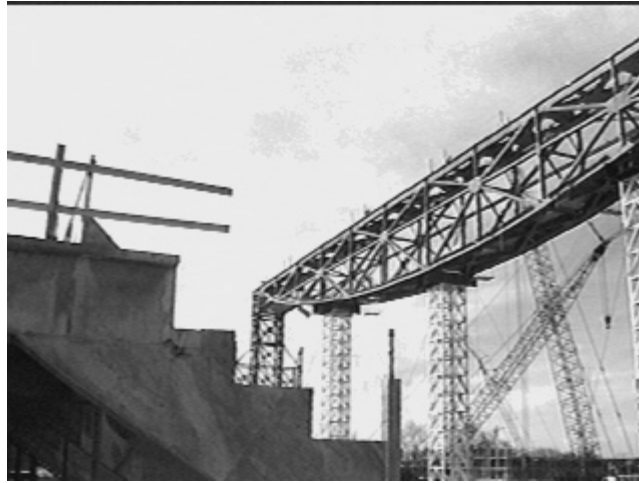
Figure 1: Georgia Tech Aquatics Center Construction
