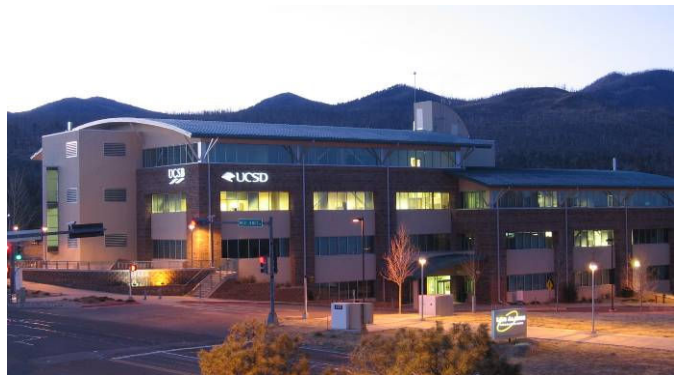
Figure 1. The Engineering Institute's facility in the Los Alamos Research Park
