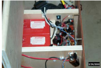
Figure 2 – Close-up of Control Compartment
