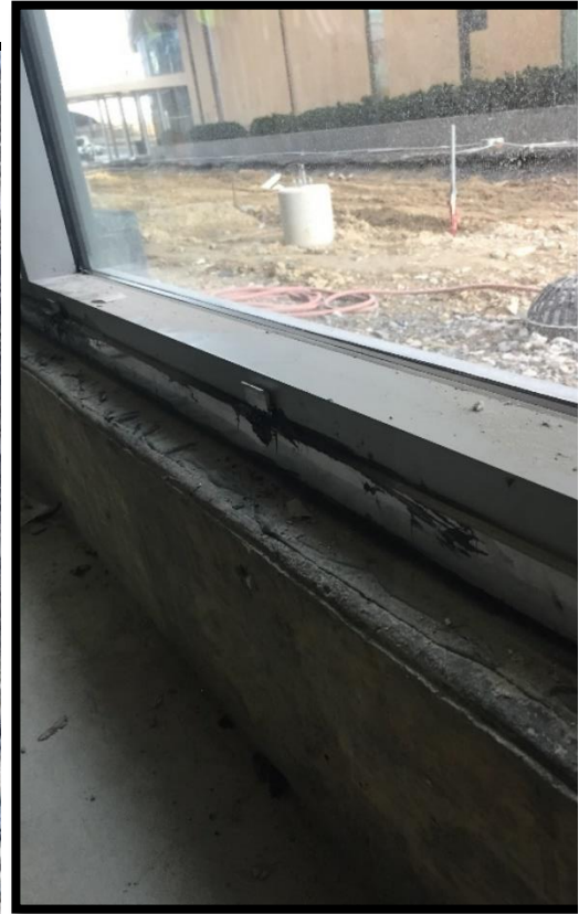
Figure A3: the underside of the exterior curtain walls
