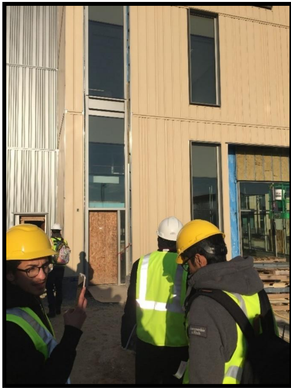
Figure A1. Picture of exterior curtain wall.
