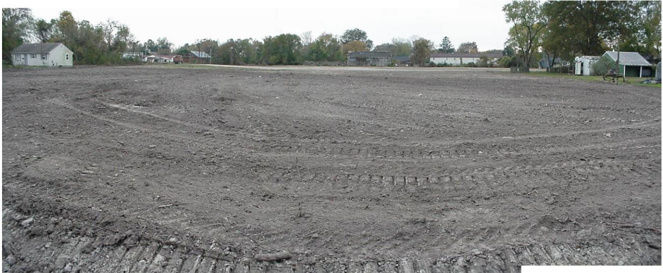
Figure 6 Completed Demolition and Site Clearance Phases
