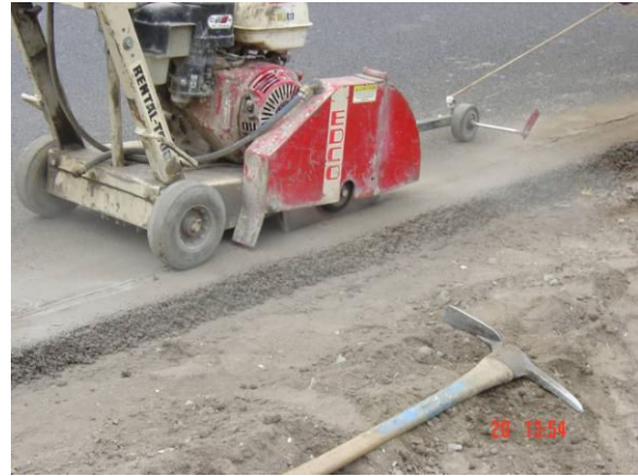
Figure 12 Final Asphalt Coat Application Figure 13 Trimming of Blacktop Edge
