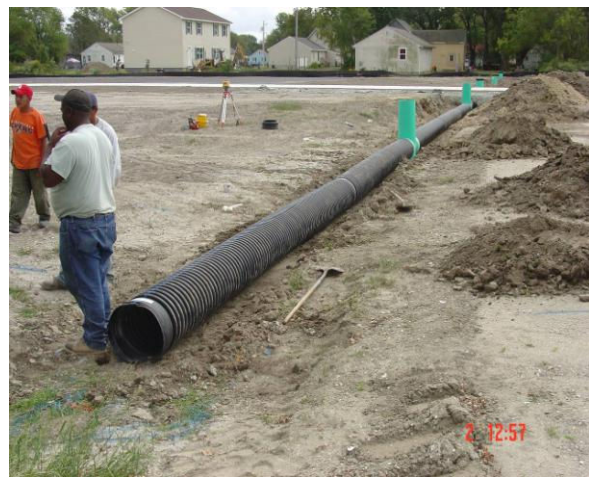
Figure 16 Construction of Walkway to the Courts Figure 17 Pipe Drainage Construction
