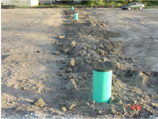
Figure 18 Drainage Inlets Before Cutting To Grade Figure 19 Final Grade
