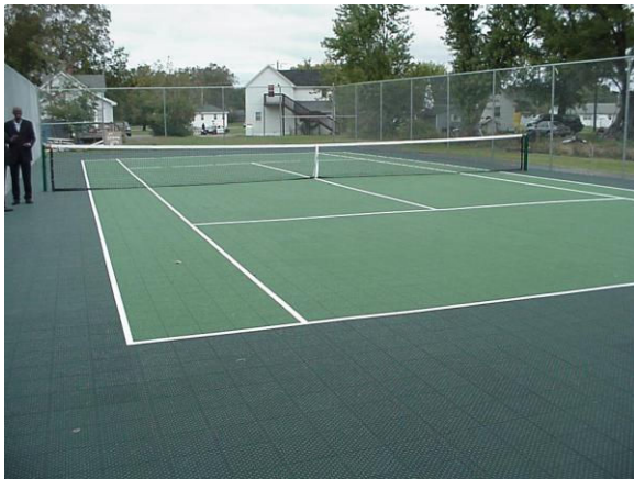
Figure 20 Finished Tennis Court
