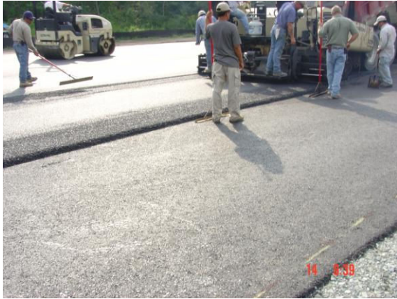
Figure 12 Final Asphalt Coat Application Figure 13 Trimming of Blacktop Edge
