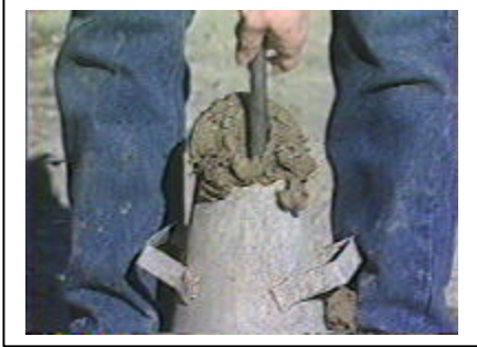
Consolidating top layer
