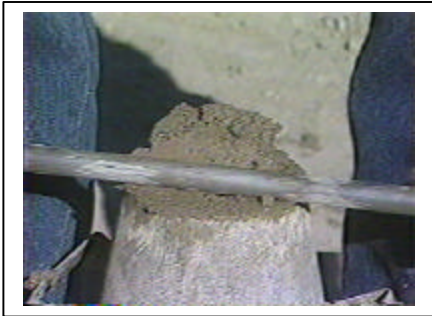
Striking off top surface
