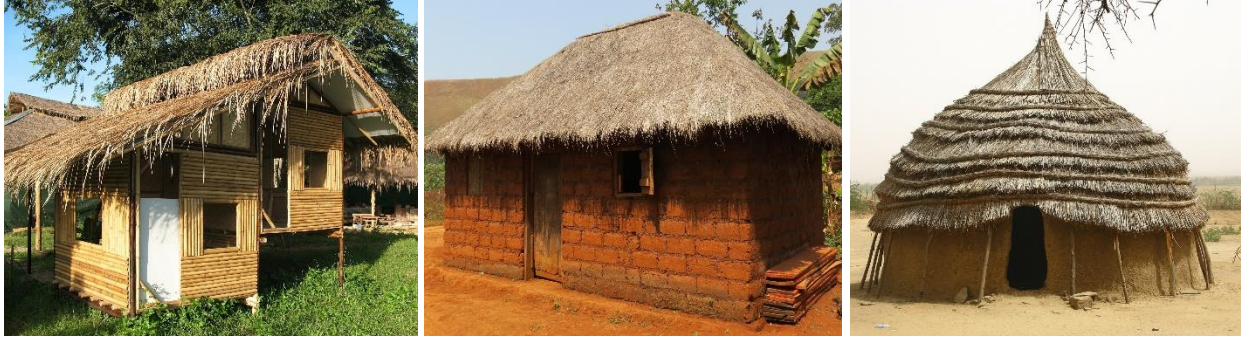
Figure 1. Examples of houses made from (left to right) bamboo, mud and straw. (Photos of bamboo and straw homes courtesy of Creative Commons licensing. Photo of mud house courtesy of Bdx.)
