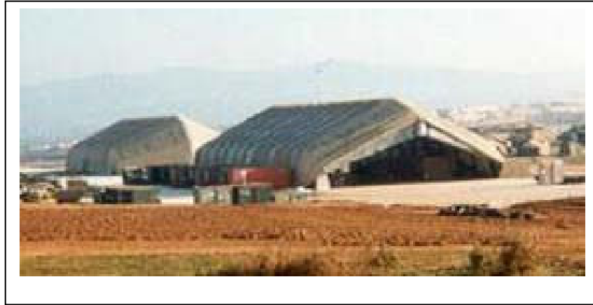
Figure 4. Photograph of a LAMS – Large Area Maintenance Shelter
