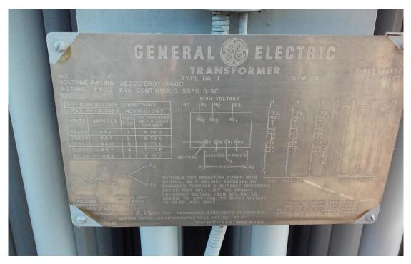
Figure 3. Nameplate of Three-Phase, 2500 kVA Transformer
