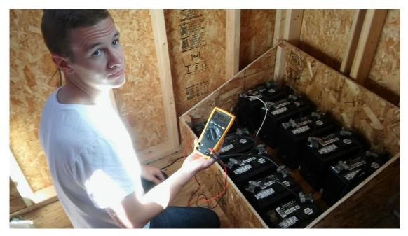
Figure 6. Testing the Control Power for the Circuit Breaker
