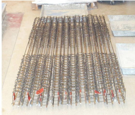
Figure 2: Twelve Reinforcing Cages Ready to be Placed in Beam Molds
