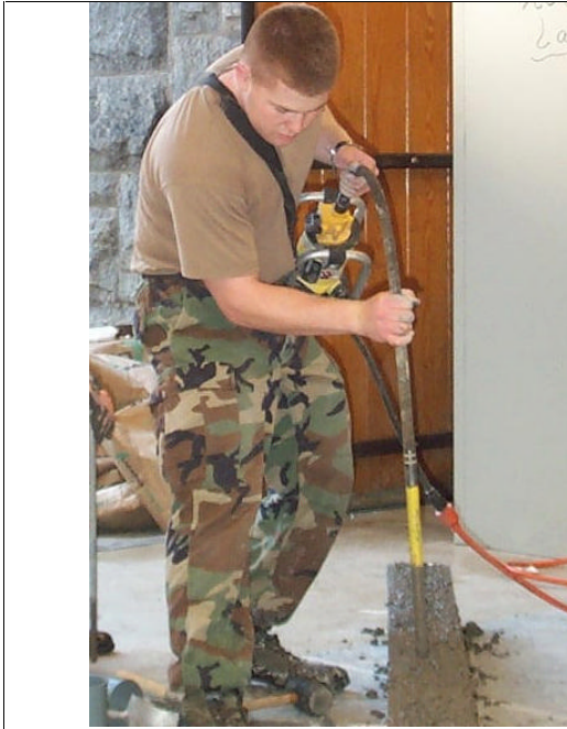
Figure 5: An Electric Vibrator is Used to Consolidate the Concrete
