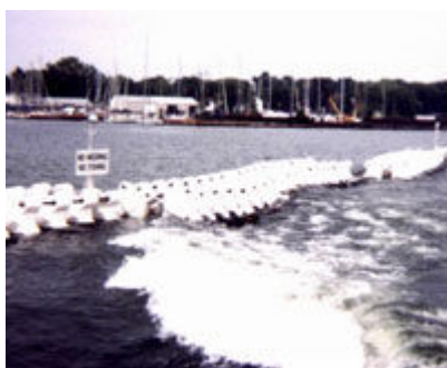
Figure 1. Floating Breakwater System (left) Consisting of an Array of Modules (right)
