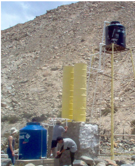
Fig. 3. Huayash solar-pumped water system sand filters.
