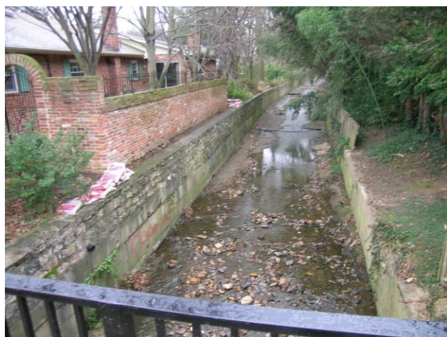
Figure 4: A section of Little Pimmit Run within the flood control project showing closeness of
