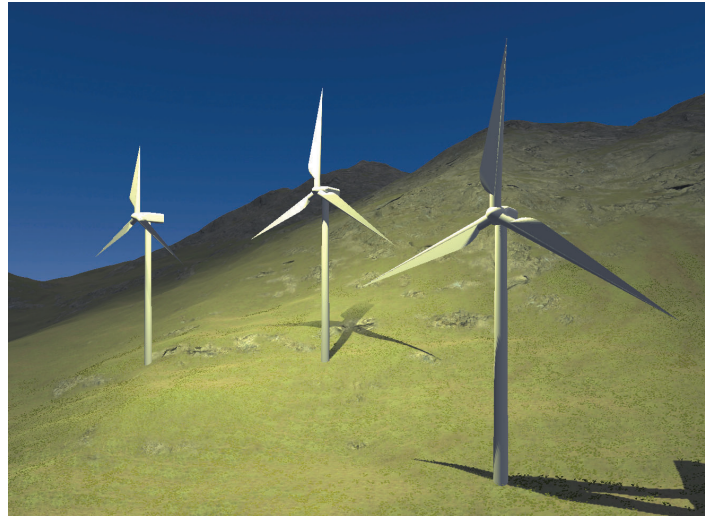
Figure 7. Wind Turbine Farm
