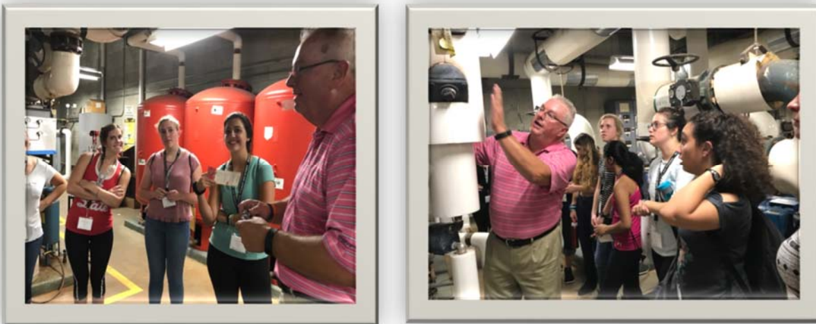
Figure 2: Photos from Schottenstein Center Mechanical Room
