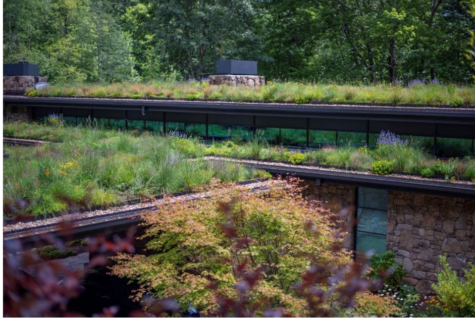
Figure 3: Sunnyland Cove is an example of a semi-intensive green roof
