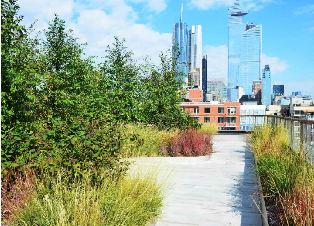
Figure 4: 510 W 22nd Street, New York is an example of an intensive green roof
