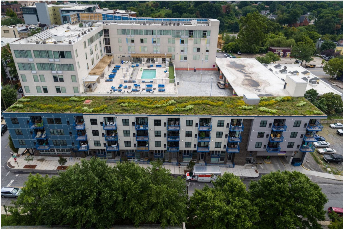
Figure 2: Example of an extensive green roof
